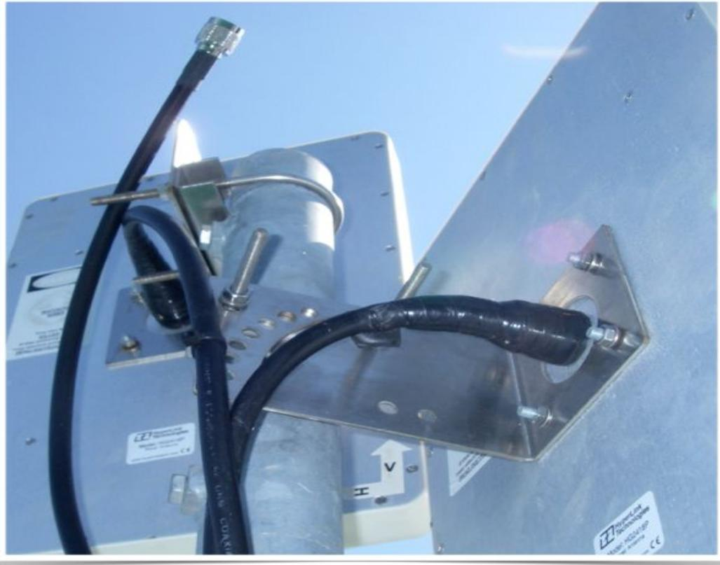
Most antenna problems are caused by coaxial cable connections that loosen due to vibration, allowing moisture to penetrate the connector interface.
